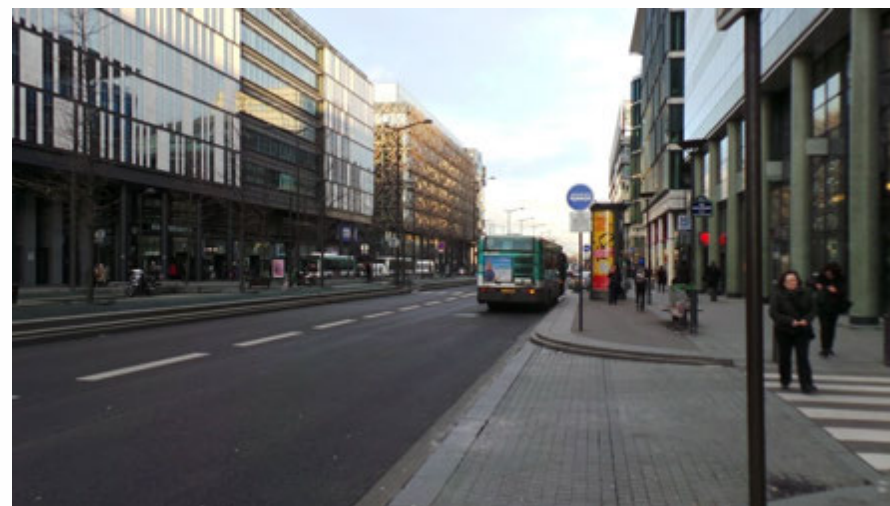
Photo existant (SNC Lavalin)
